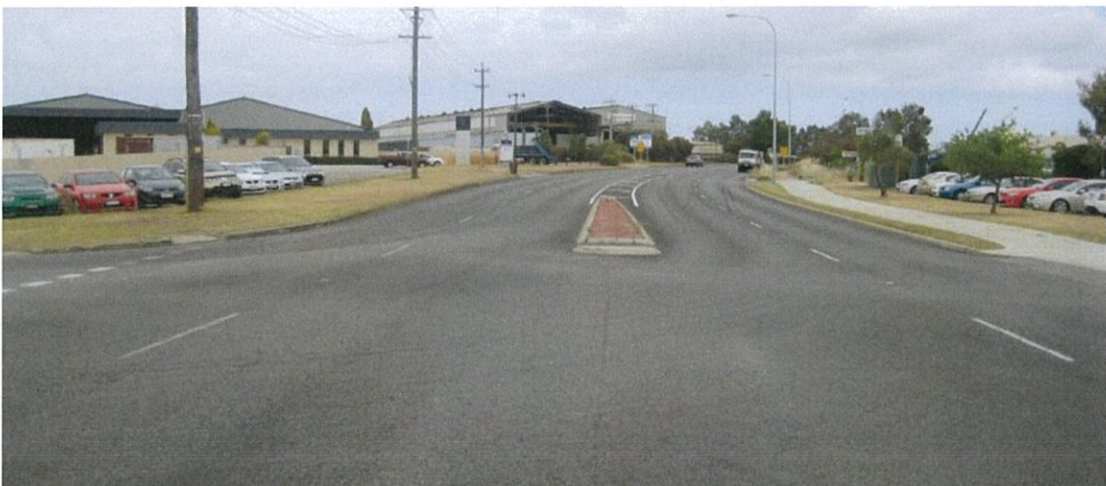
Figure 6: Collier Road looking west in the vicinity of the development site
